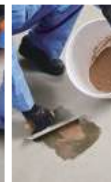
(4) Apply using plastering brush, pushing in (lower than level of subfloor)
