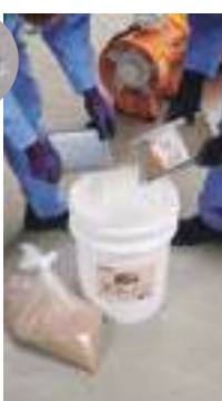
(2) Mix solution A and B by weight (always use a mixer)
