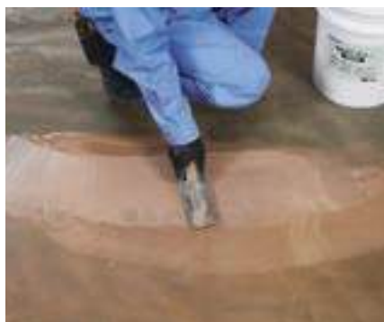
After applying Dynamic load resistant floor Primer, apply using a plastering brush, rubbing into subfloor.
