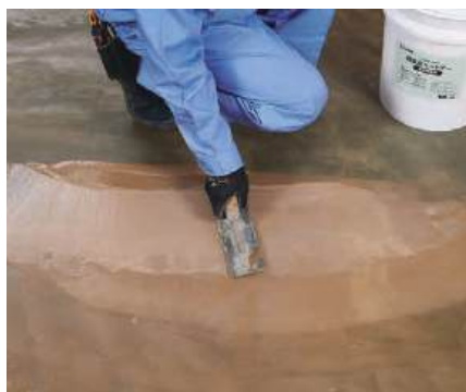
After applying Dynamic load resistant floor Primer, apply using a plastering brush, rubbing into subfloor.
