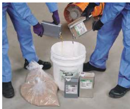
Mix solutions A and B by weight (always use a mixer)
