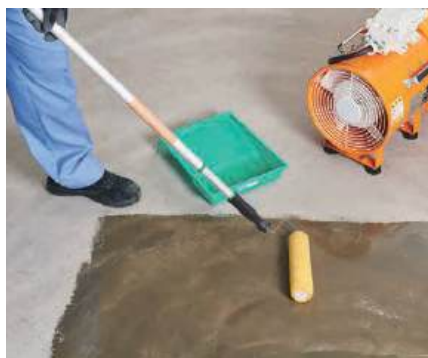
Apply using a roller brush. Always use ventilation fans (explosion-proof type) while applying.
