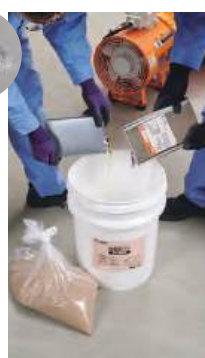
(2) Mix solution A and B by weight (always use a mixer)
