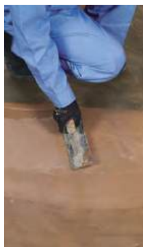
(5) After Dynamic load resistant floor Primer dries, apply Dynamic load resistant floor Hardener
