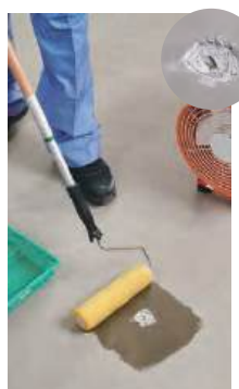
(1) Apply Dynamic load resistant floor Primer
