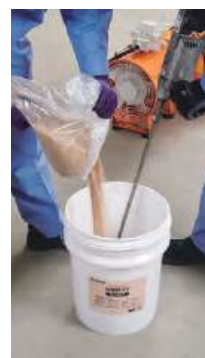
(3) Mix in aggregate (always use a mixture)
