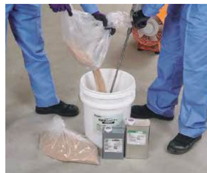
Mix in aggregate (always use a mixer)
